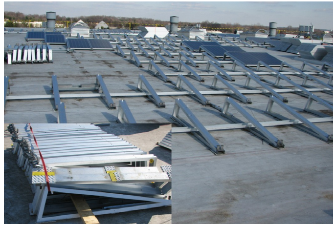
Racking system for the panels on the roof, inset showing the contact points of the rack with the roof membrane compatible wear pads.
