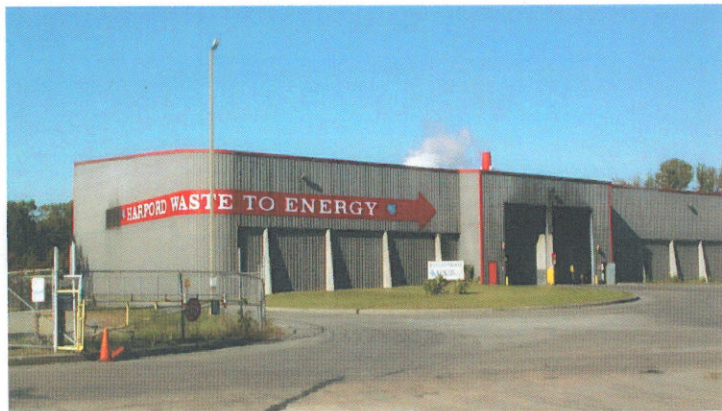
Harford County Waste-to-Energy Facility in Joppa, MD
